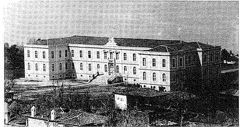
1. The idadî school of Trabzon. Note the classical style of the building, and the Black Sea in the background. (Source: Istanbul University Rare Book Library)
